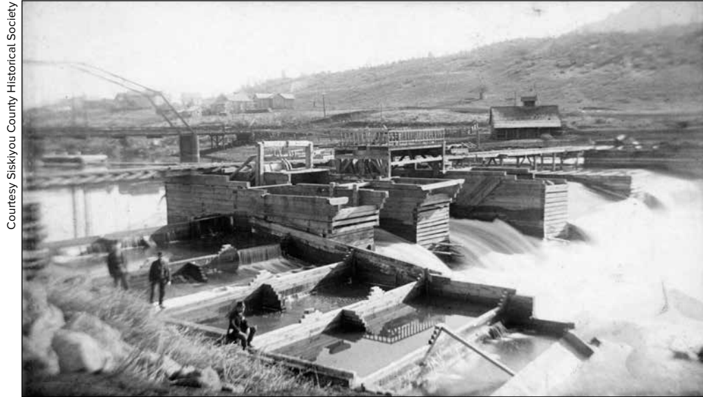
THE REBUILT KLAMATHON MILL log-crib dam and fish ladder is pictured here in 1892. The original 1889 dam did not provide a path for fish passage, and many salmon died downstream or were captured and illegally sold.
