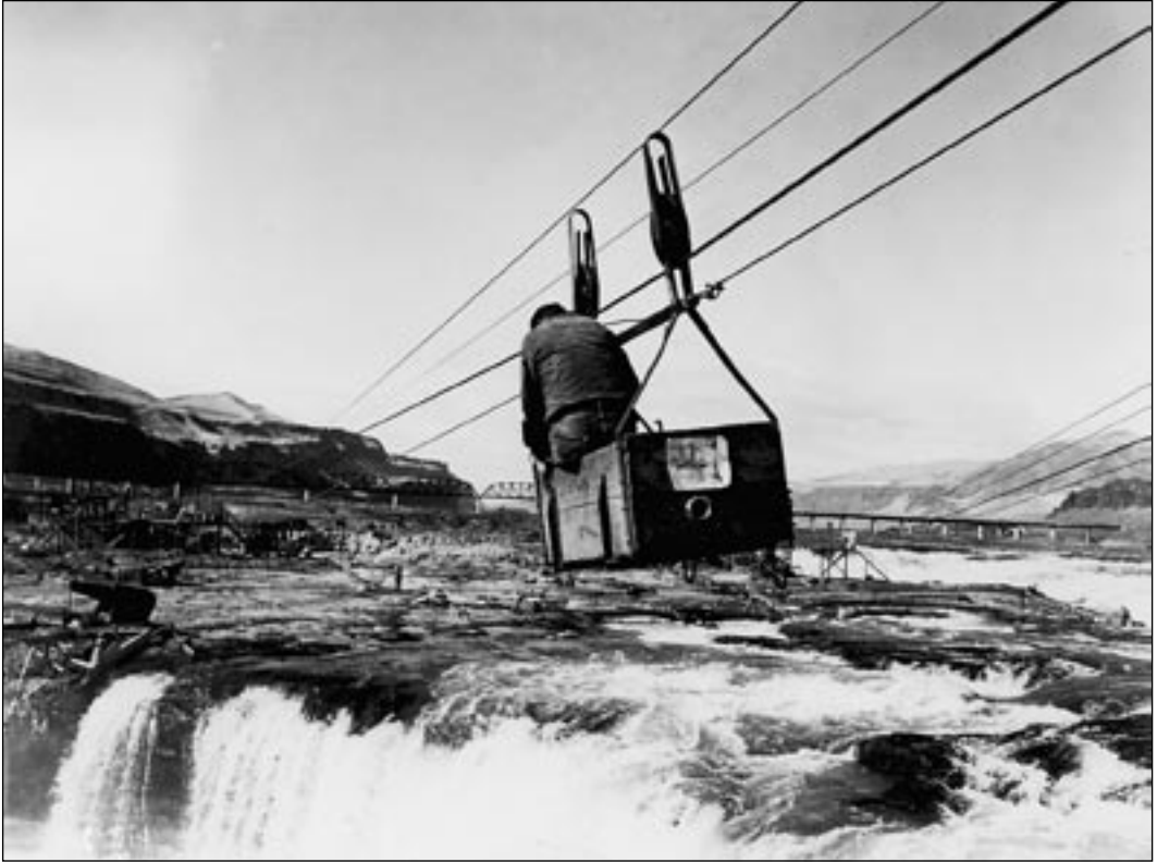
Before Seufert Brothers Company installed the first cableway at Celilo Falls in 1930, fishers reached their stations by canoe. The new aerial routes helped attract a horde of newcomers to the falls during and after the Great Depression. This 1951 photograph shows a fisher using a motorized cableway between the Oregon shore and the islands at the falls.
